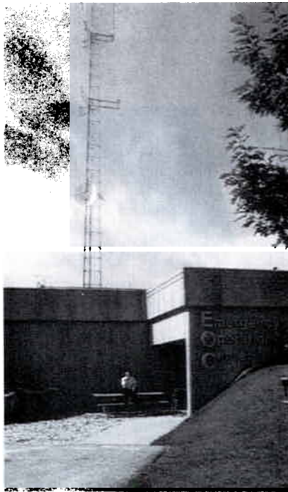
The Carroll County, Maryland, Communications Center was severely damaged by lightning in 1987. Installation of a Teleline Isolator effectively protected their equipment and personnel.
