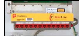
Fig 11: 7250BB-50 Break-Out Box installed on 720000 TeleLite Shelf
