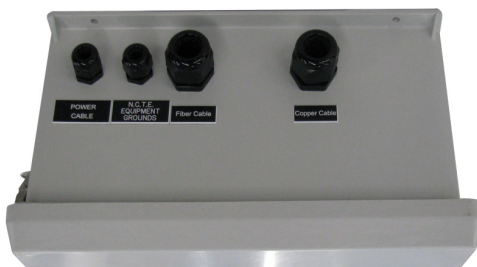
Engraved plates identify cabling entrance and exit. Vapor-tight strain relief provided for cabling.
