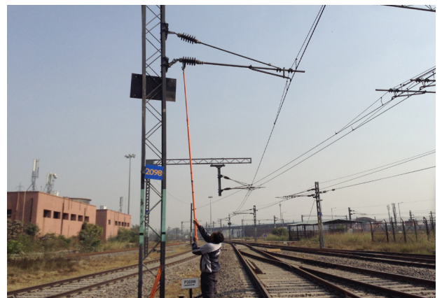
Testing 25kV Post Insulators in Railways
