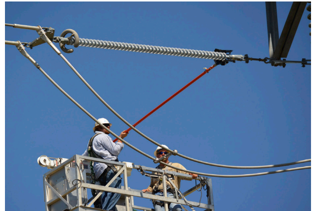
Testing Polymer Insulators on 345kV HV Line
